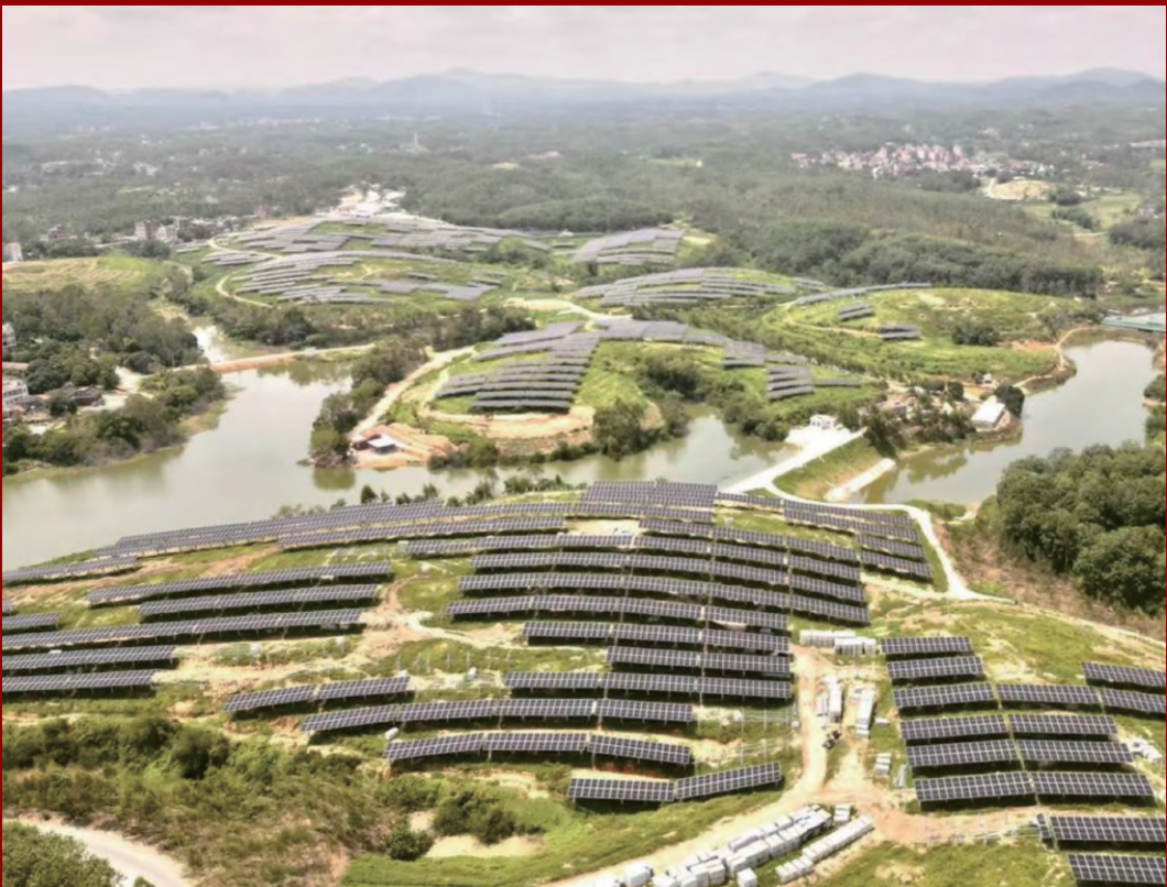
Solar power stations are set up in rural areas to provides clean electricity to local farms while reducing carbon emissions.
